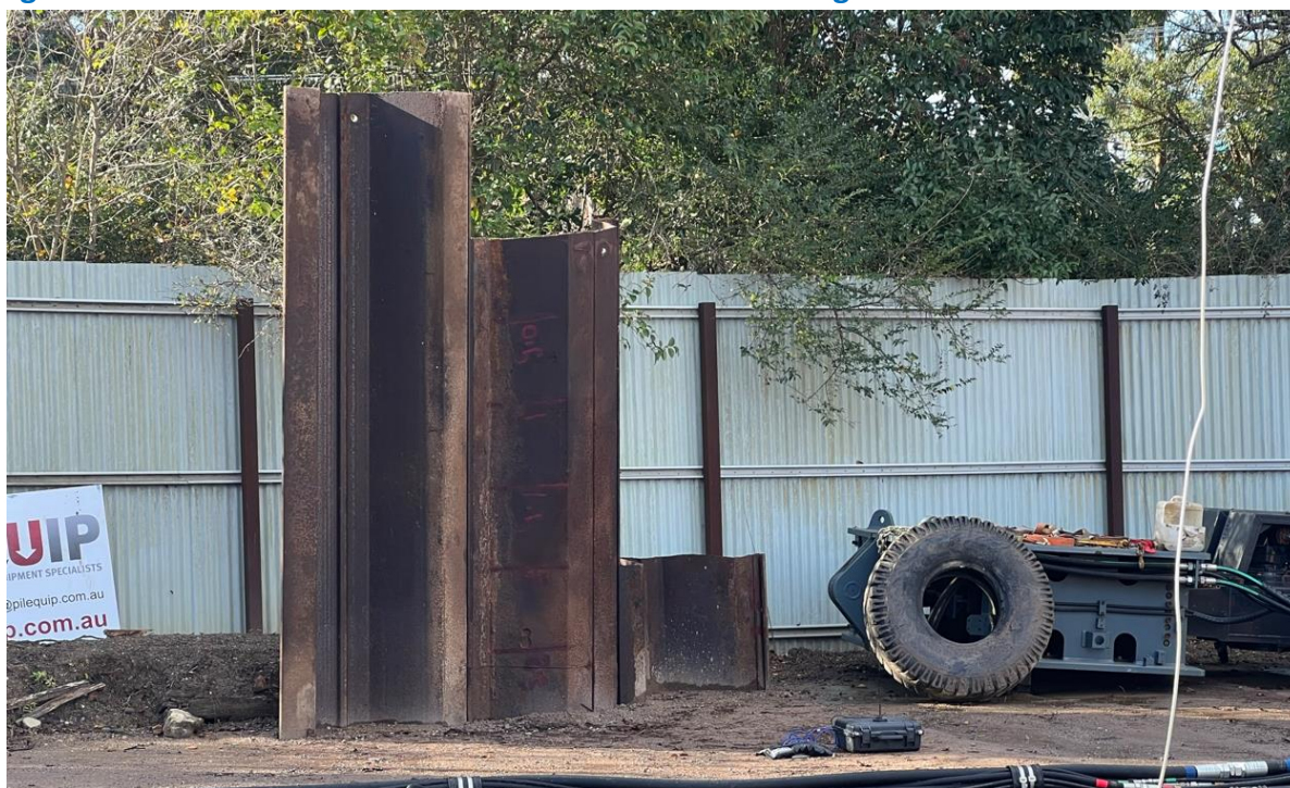
Figure 3 Photo of Double Z Sheet Piles Used in the Testing
